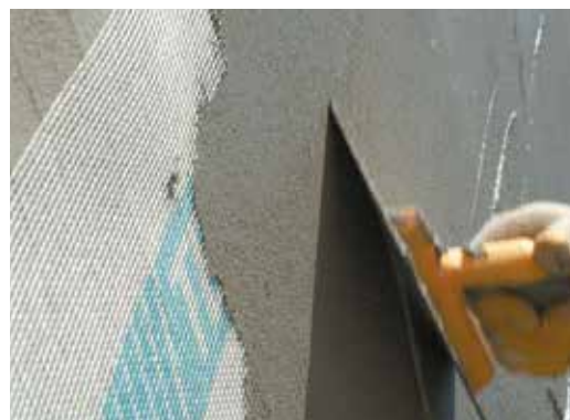
Embedding Glass Fibre Mesh
