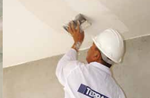
Levelling Sprayplaster™ FC with spatula
