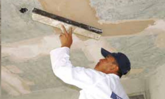
Applying Sprayplaster™ BC at joints
